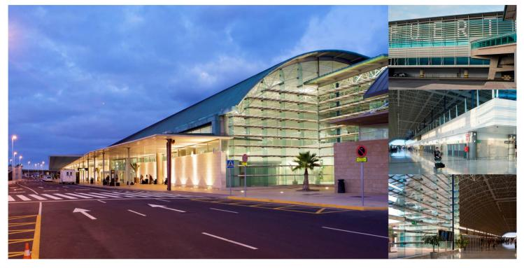
At Fuerteventura Airport all the floors have been solved employing exclusively two expansion joints (axis 11 and 23), which divide slab surface areas of approximately 132.0m x 62.0m and 144.0m x  $62.0m^2$ . To fulfill this operation a special study regarding the reinforcement was undertaken.
